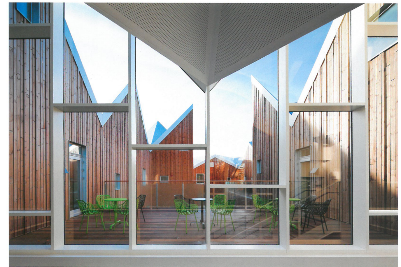
Vlietland Ziekenhuis, Schiedam, the Netherlands, EGM Architects, 2008. The generous lobby and reception space with its wooden ceiling creates a welcoming atmosphere for patients and visitors.
