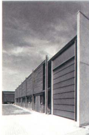
Exterieur techniekhallen Exterior technical halls
